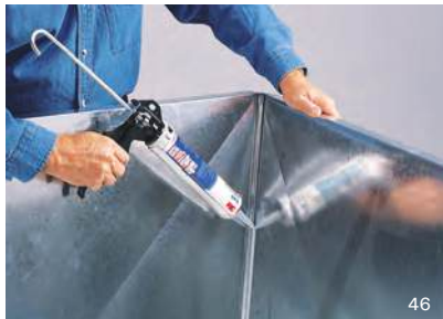
Seam sealing ductwork with 3M™ Polyurethane Sealant 540 will prevent air and dust intrusion. Its flexibility assists with vibration damping.
